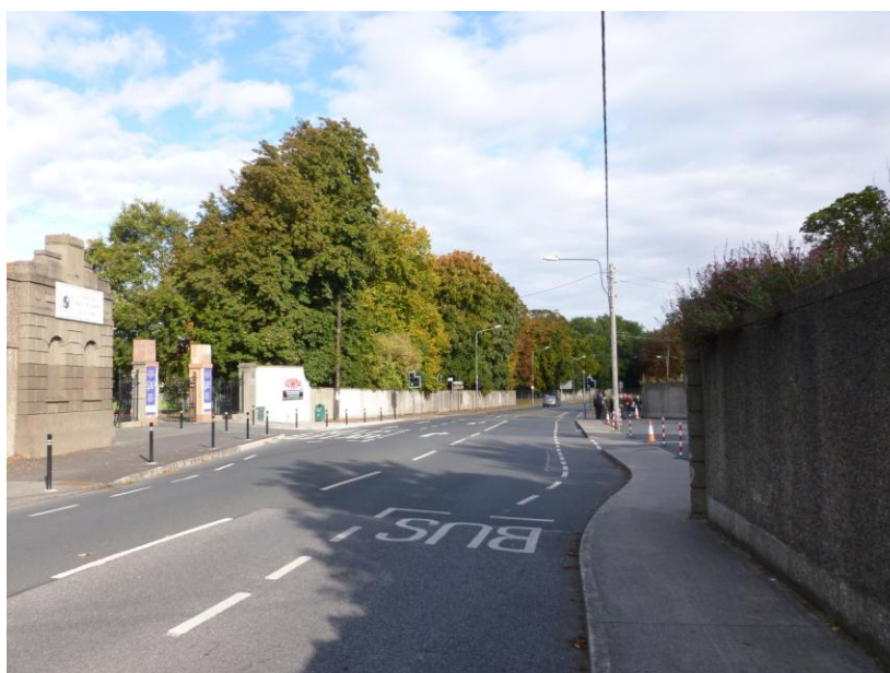
Plate 3.2 Road carriageway and entrances categorised as BL3 south of Dispensary Lane close to Loreto Abbey.
