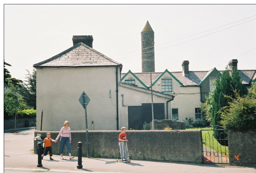
16 TOWER ROAD FROM THE NORTH
