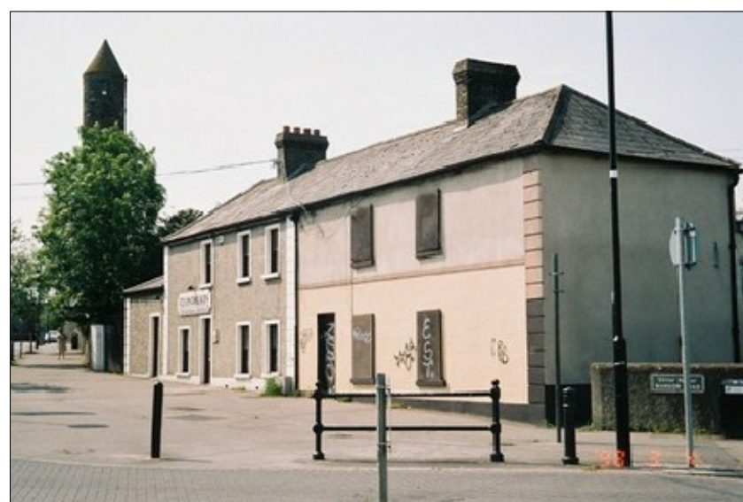
15 AND 16 TOWER ROAD FROM THE NORTH
