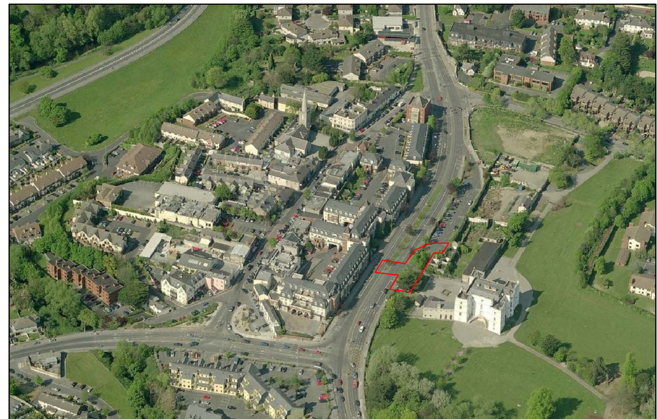
02 AERIAL VIEW OF RATHFARNHAM VILLAGE SITE FROM THE SOUTH P8 SOURCE: BINGMAPS.COM
