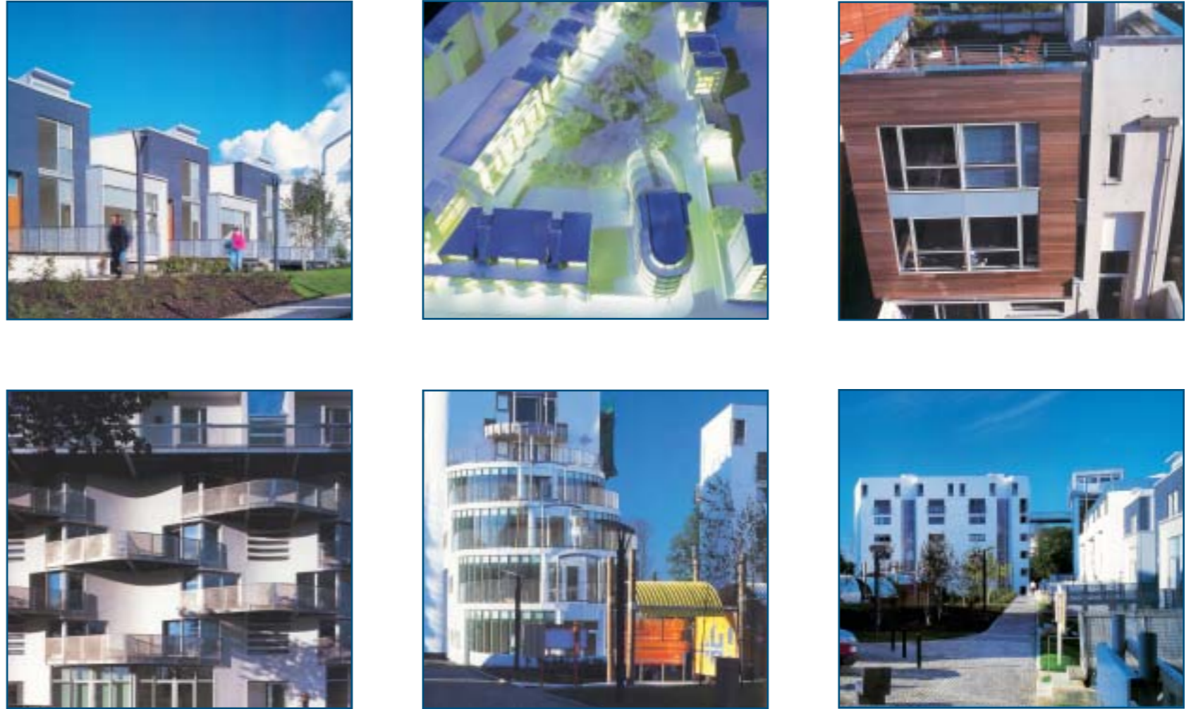
Figure 2.16. Variety of Modern Building Forms and Styles, 'Homes for the Future' Demonstration Project, Glasgow
