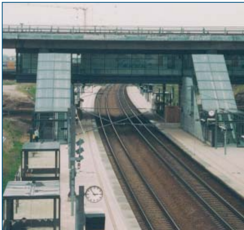
Figure 2.23. Railway Station/Transport Interchange
