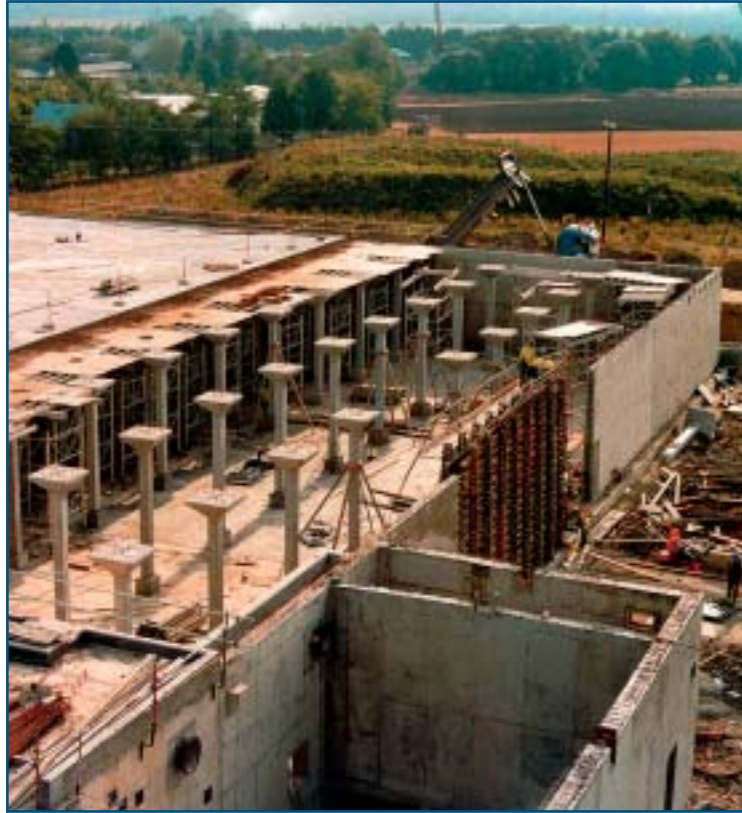
Figure 2.31. Peamount Reservoir Under Construction (Lucan - Palmerstown High Level Water Supply Scheme)
