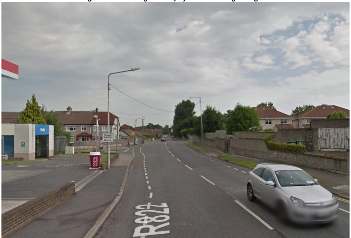
Figure 2.7 : Grange Road immediately north of Barton Drive
