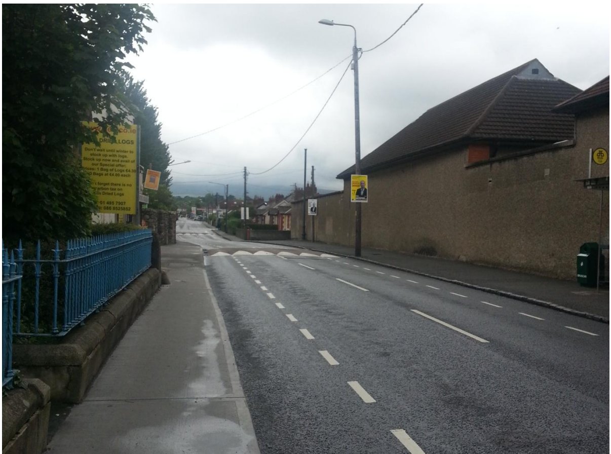
Figure 2.8 : Existing traffic calmed section of Grange Road
