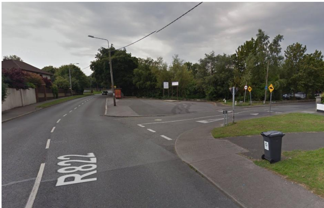
Figure 2.5 : Junction of Grange Road/ Sarah Curran Ave/Barton Drive (Google Streetview)
