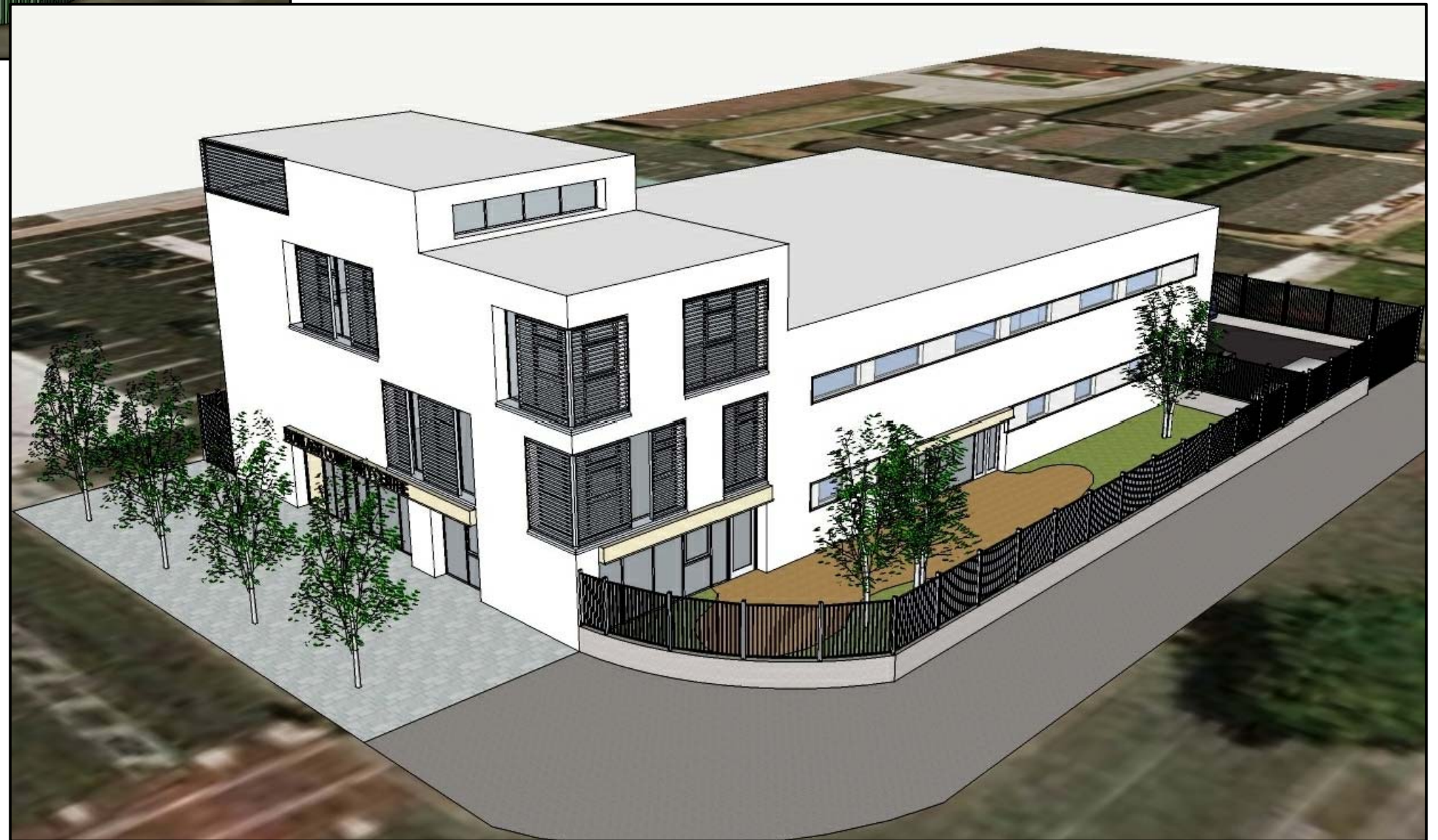
AFTER VIEW FROM NEILSTOWN ROAD APPROACHING FROM CLONDALKIN EXISTING BUILDING NOW CLAD IN RENDERED INSULATION AND PAINTED TO SELECT COLOUR, NEW 3 STOREY EXTENSION REPLACES LEAN-TO EXTENSION. RAILINGS REMOVED FROM FRONT OF BUILDING TO PROVIDE WELCOMING RECEPTION FROM NEW PLAZA AREA. NEW LOW WALL WITH PAINTED GALVANISED FENCE TO ENCLOSE PRIVATE GARDEN FOR CHILDCARE FACILITY AND PRIVATE CAR-PARK TO REAR
