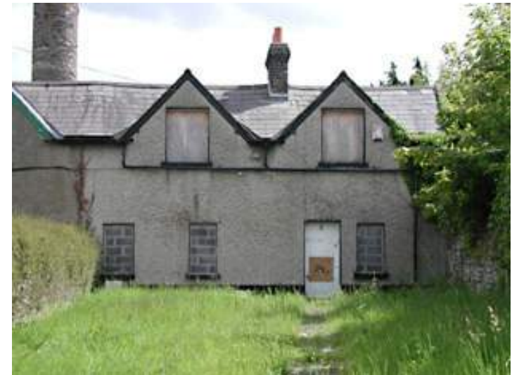
Plate 6 Western end of Millview Terrace (AH1), viewed from north. Round tower in background.
