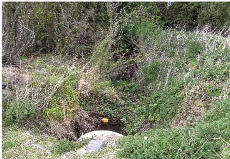
Plate 4: View of culverted drainage ditch
