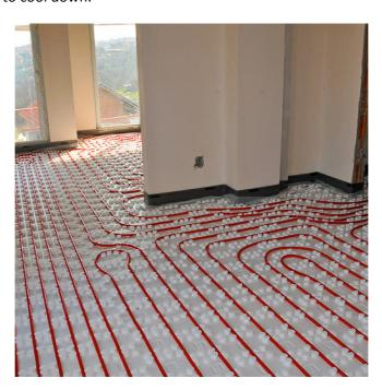
Image 1- Underfloor Heating Pipework Before Screed Pour
