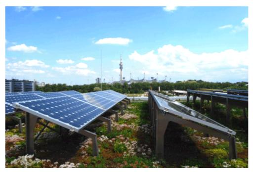
Image 8 - PV Panels on a Green Roof
