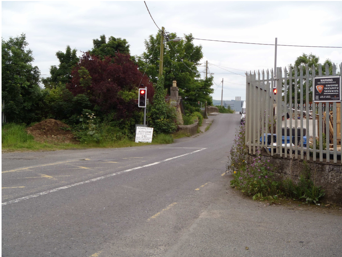
Fig 5. Trees around garden on NE side of bridge – potential bat feeding area
