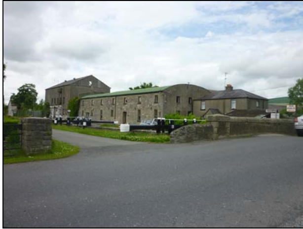
Plate 17 View to mill buildings to the northwest of Leck Bridge
