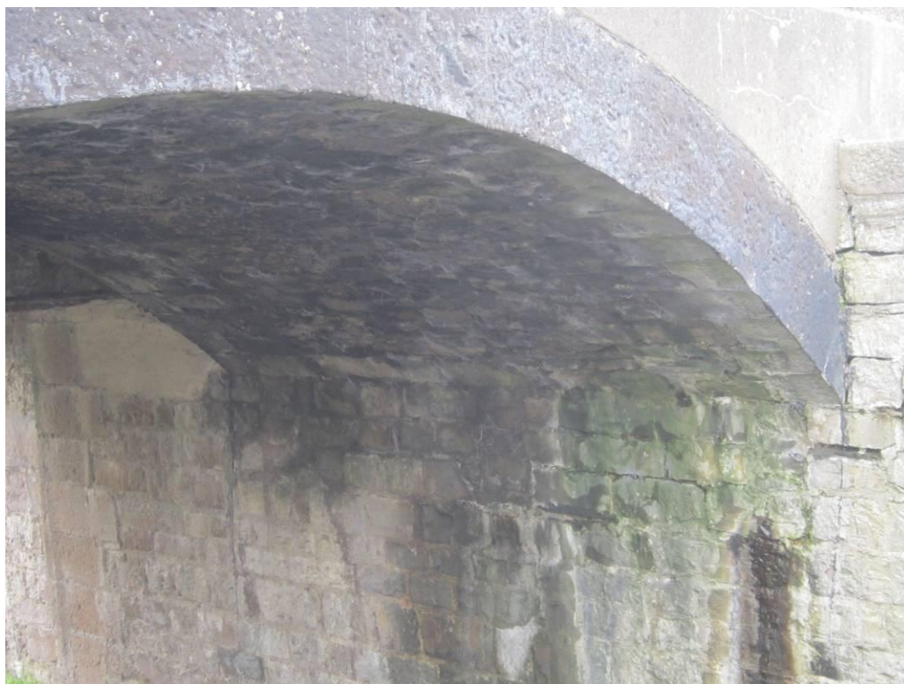
Photograph 11: Soffit of Arch Barrel
