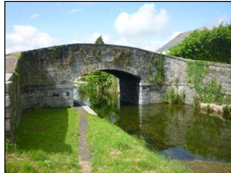
Plate 24 Canal bridge at Hazelhatch
