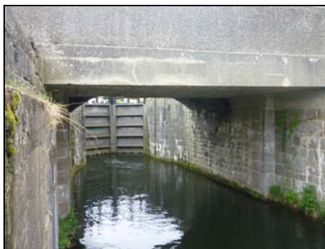
Plate 10 Flat arched concrete extension to bridge
