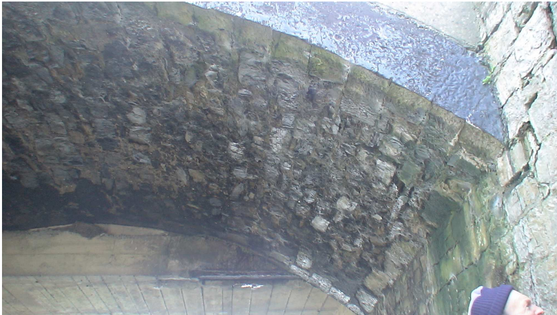
Fig. 6. Stone-arched section (1775) of bridge with potential cavities for Daubenton's bat
