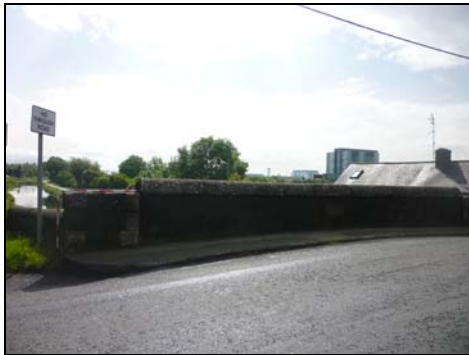
Plate 12 Eastern bridge parapet from the west
