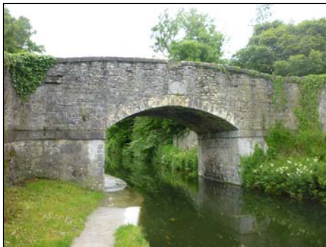
Plate 23 Canal bridge at Lyons Estate
