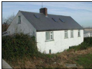
Plate 5 Rear of structure (2006)
