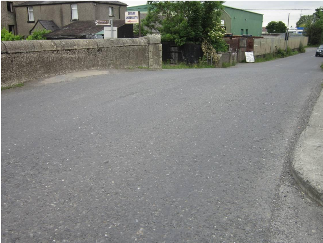
Photograph 1: General View of Carriageway Surfacing
