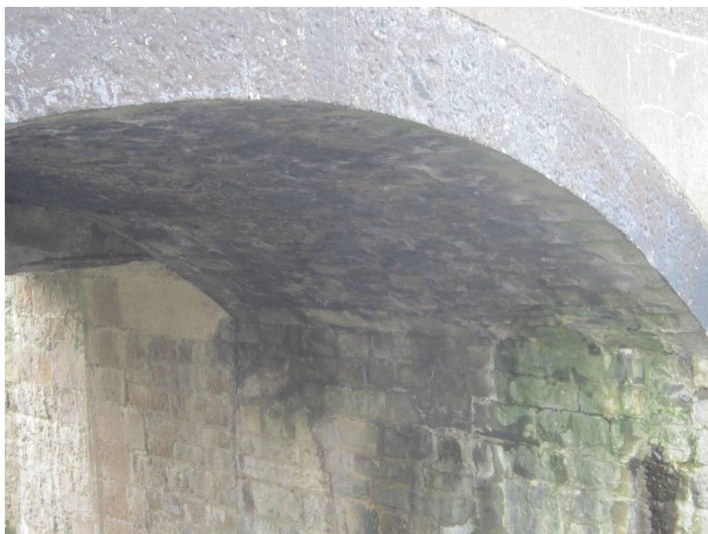
Photograph 13: Spalling on Edge of Concrete Deck
