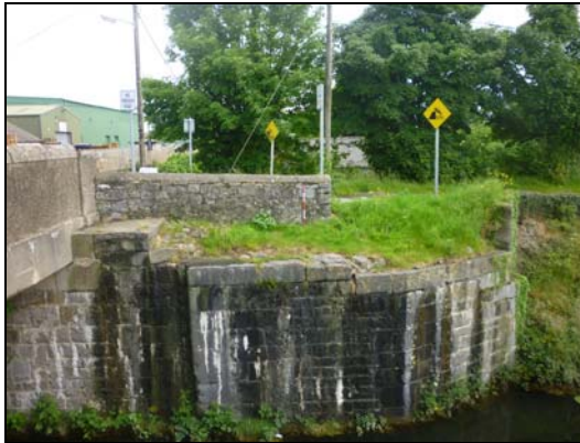
Plate 15 Northern lock wall, east of the Leck Bridge
