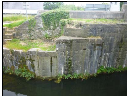
Plate 16 Southern lock wall, east of Leck Bridge
