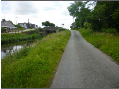
Plate 19 Tow path to the north of the canal, east of bridge
