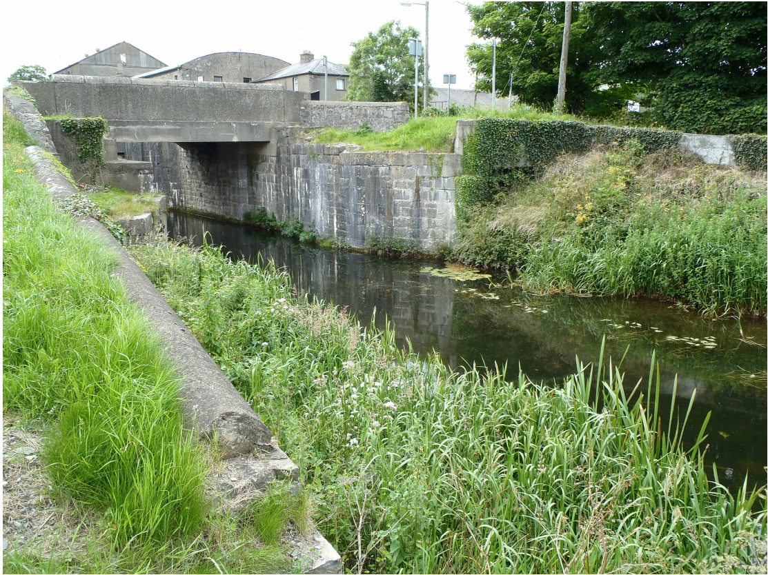
Fig. 2. Northern side of Canal at bridge widening site
