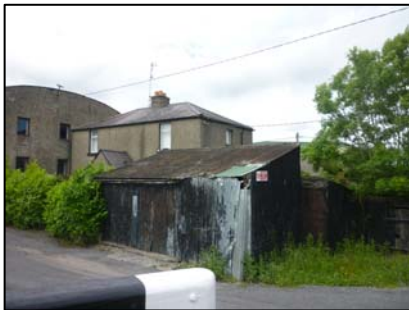
Plate 18 View from the east to a two story structure with associated corrugated iron sheds, fronting onto the canal.
