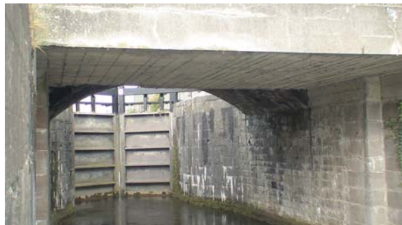
Figure 3.4 – Underside of 1932 bridge extension
