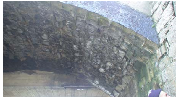
Figure 3.5 -Underside of 1770's Arch Structure
