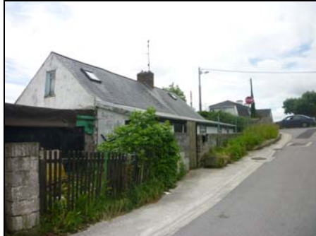
Plate 3 Structure taken from the northeast (ID4)
