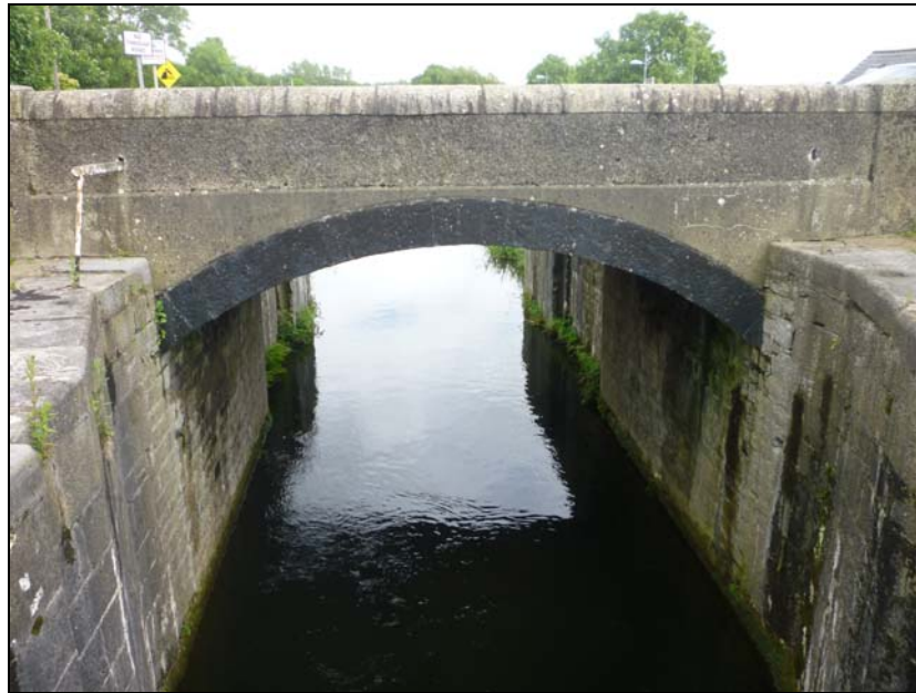
Plate 8 Original arch, west side of bridge, dating to c.1770
