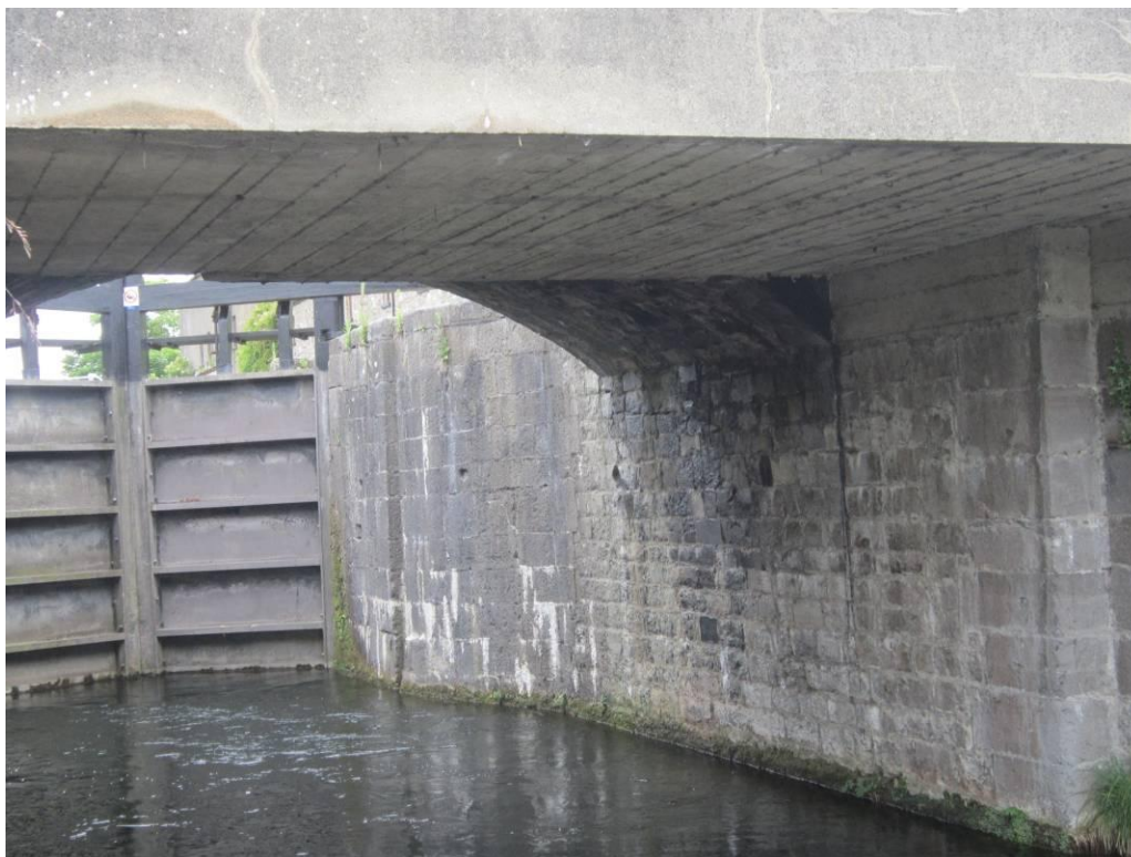
Photograph 12: Soffit of Concrete Deck
