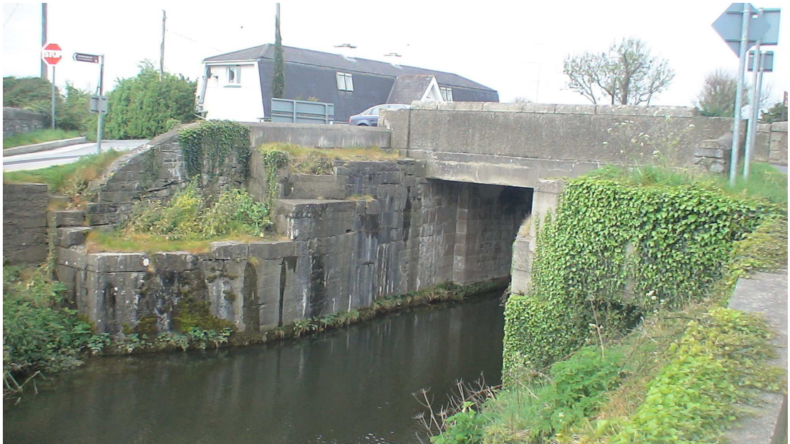
Fig. 3. Southern side of Canal at bridge widening site
