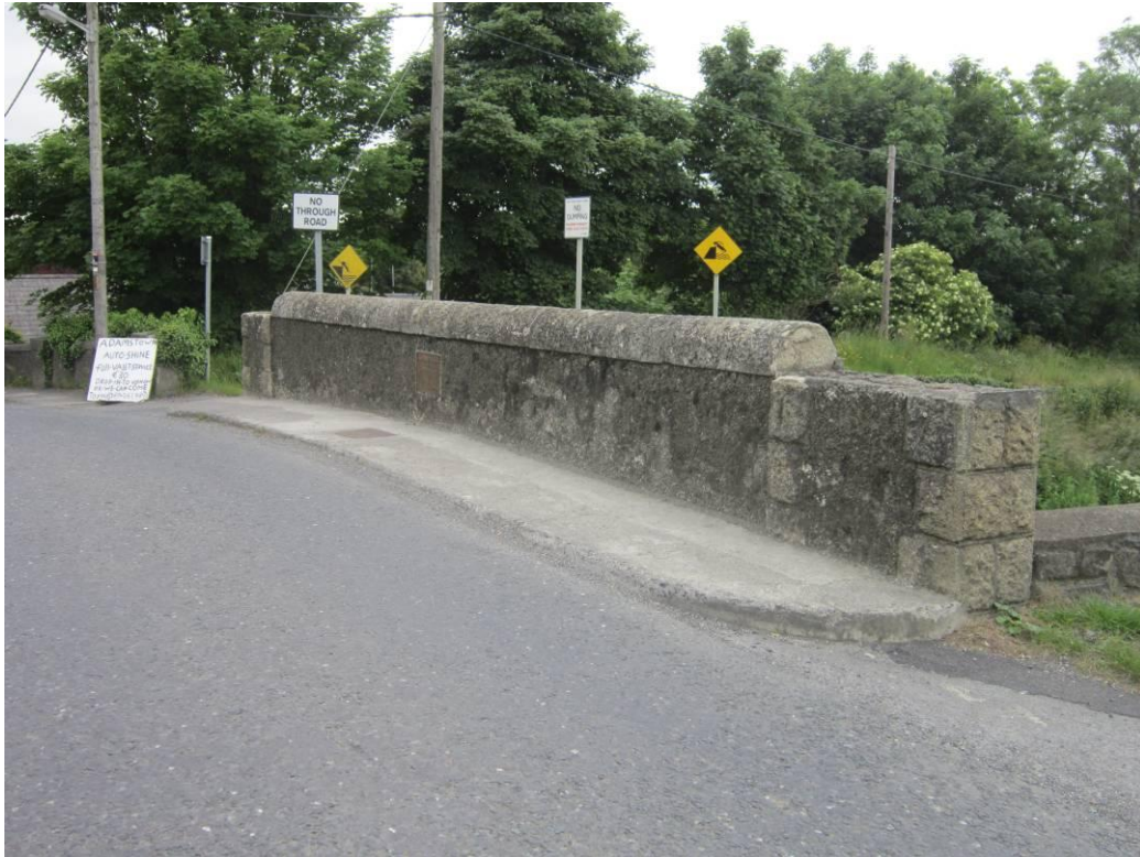
Photograph 4: East Footway and Parapet
