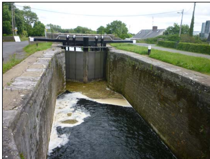
Plate 14 The 12 th lock chamber taken from the west
