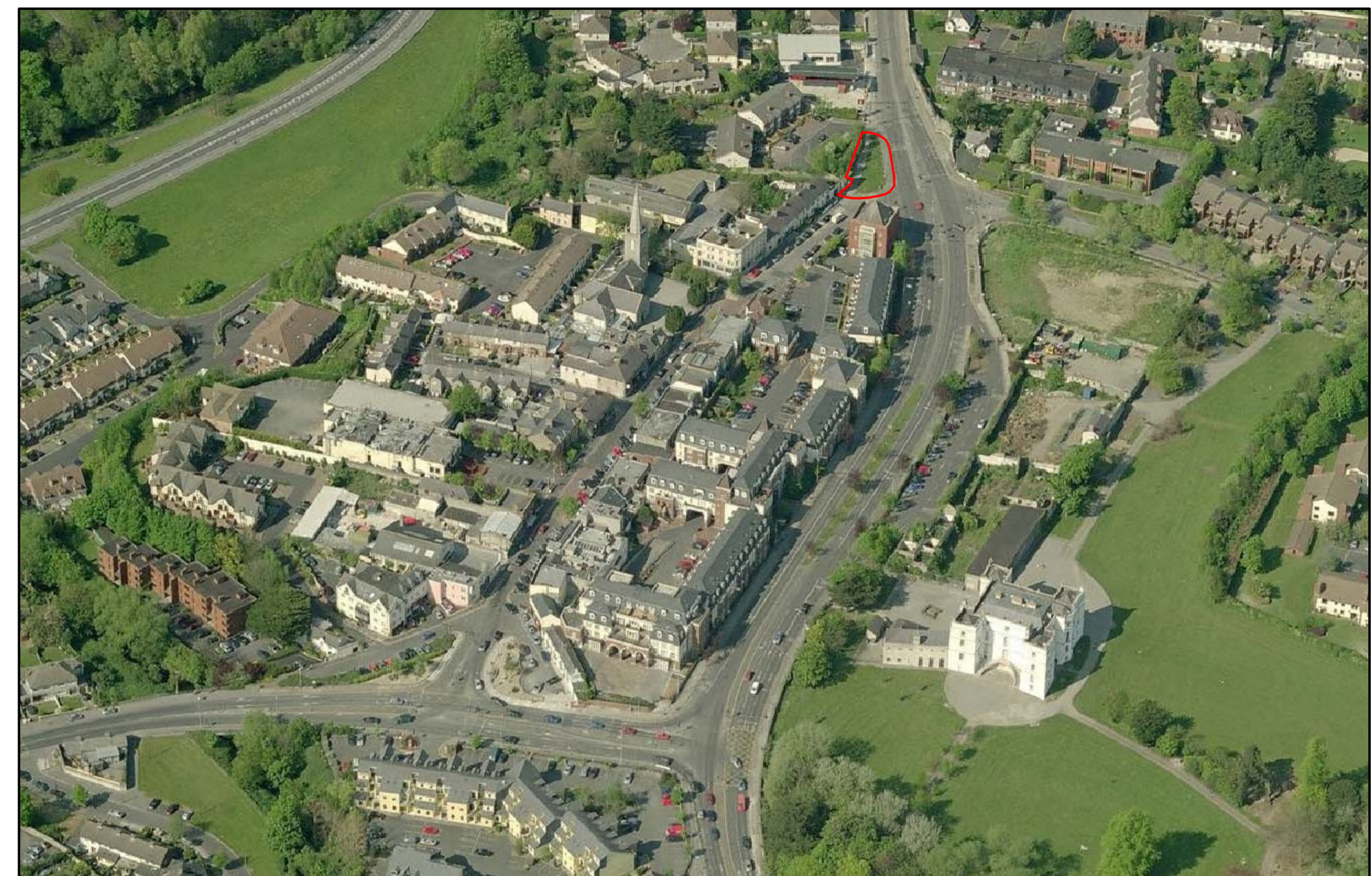
01 AERIAL VIEW OF RATHFARNHAM VILLAGE SITE FROM THE SOUTH P8 SOURCE: BINGMAPS.COM
