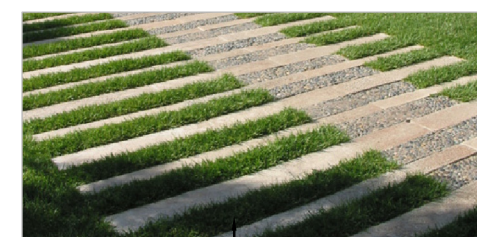
Grass graded into landing of resin bonded surface
