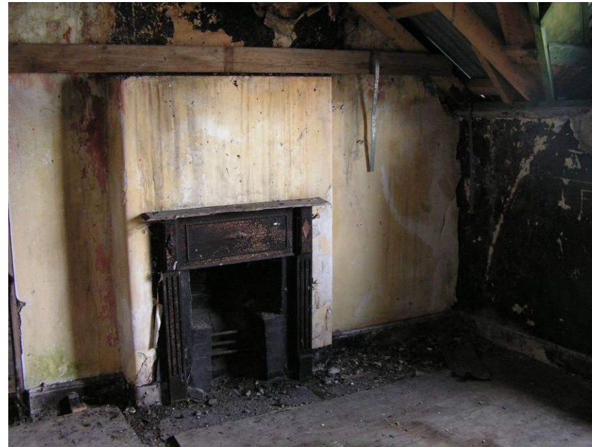
Fig. 11.10. A cast iron Edwardian surround in 1 Millview Terrace, at first floor level. (March 2013)
