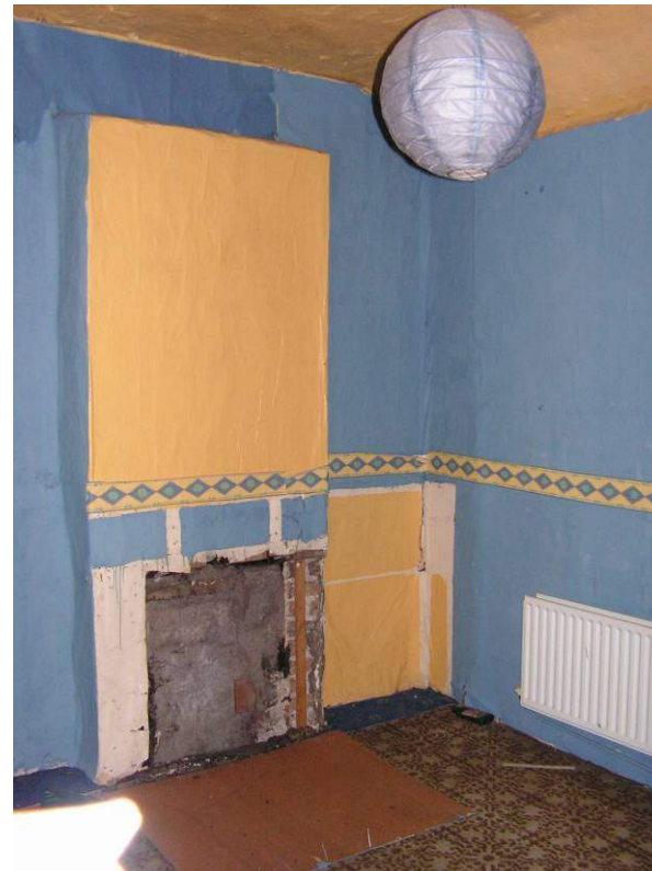
Fig. 6.19. 16 Tower Road: first floor bedroom. (January 2014)
