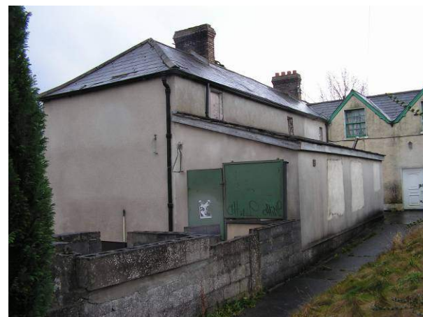
Fig. 6.3. The extension to 16 Tower Road which occupies most of the former yard space of number 16, as shown in the 1969 ordnance survey map (Figs.4.84D, pg. 65 and 4.78, pg. 62). (January 2013)
