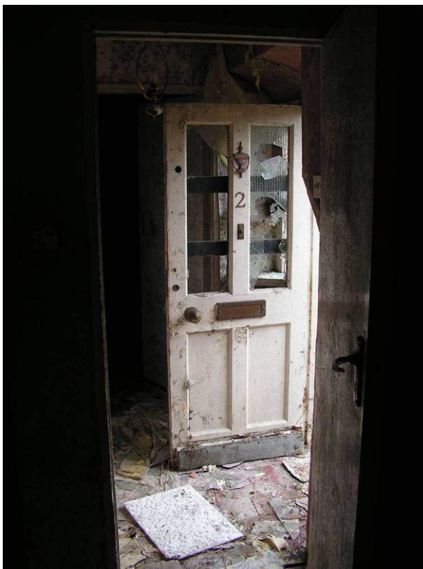
Fig. 7.12. The front door to 2 Millview Terrace. (March 2013)
