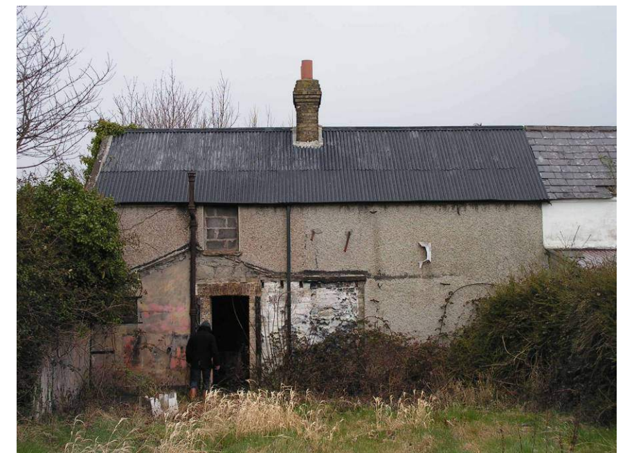
Fig. 8.2. The rere façade of 1 Millview Terrace. The outline of the demolished extension on the rere façade is clear. The side wall of the extension remains on the left side of the photo, just inside the boundary wall which is concealed in the hedge further to the left. (March 2013)
