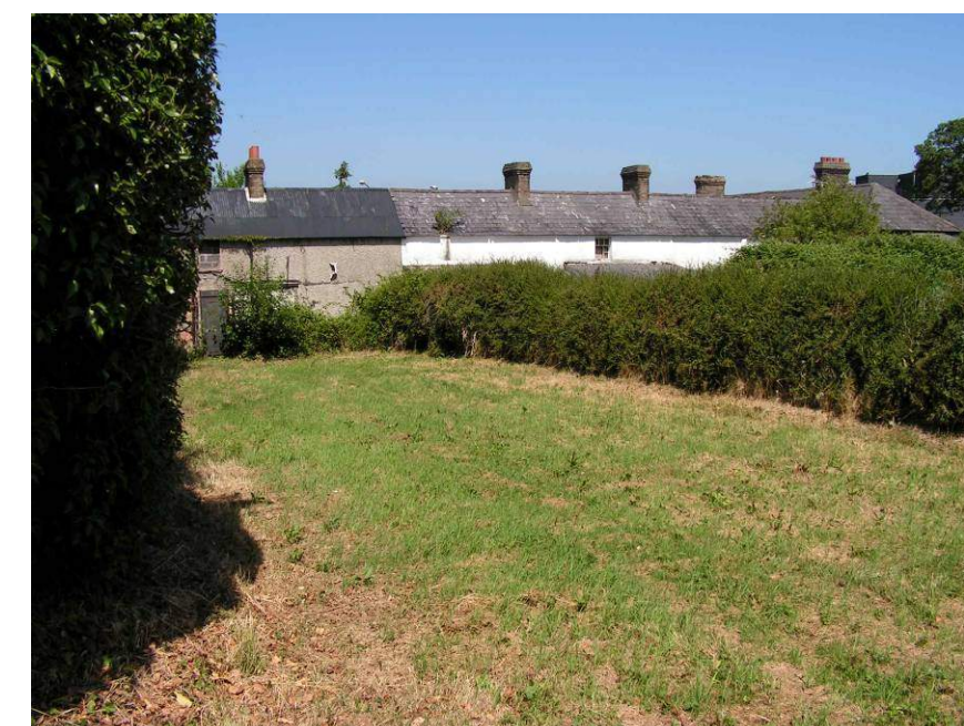
Fig. 1.7. The backs of 1, 2 and 3 Millview Terrace (from left to right) and the hipped roof of 15 Tower Road on the right viewed from the south.
