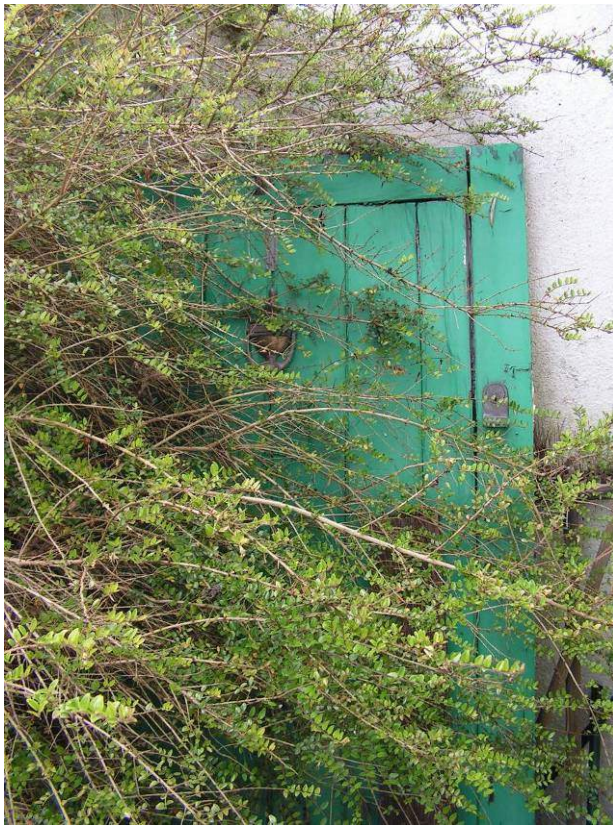
Fig. 7.11. 3 Millview. The door was stored in the back yard. (May 2011)
