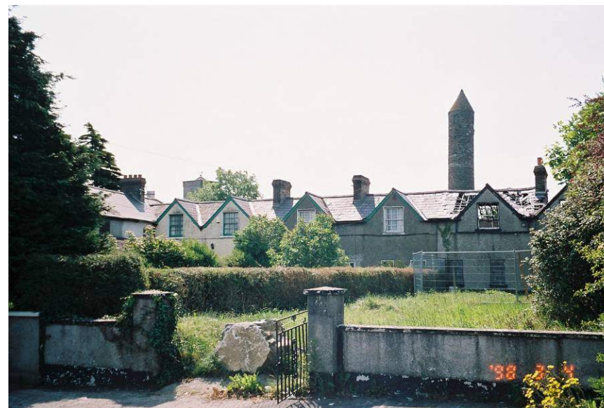
Fig. 8.5. A view of the fronts of the houses at Millview Terrace, May 2007 (the date on the bottom right corner of the photo is incorrect). The fire-damage to the roof of number 1 is visible. This has since been stripped and re-covered with a new corrugated sheet on a new roof structure. Note the absence of any breaches in the roofs of numbers 2 and 3 and the general good appearance of the front windows; the condition of these roofs and windows have deteriorated rapidly in the 7 years since this photograph was taken. Neglect and vandalism are the causes. Compare this view with more recent views on Figures 7.3 and 7.5 on page 79. (Photo courtesy of South Dublin County Council's Architectural Services department)
