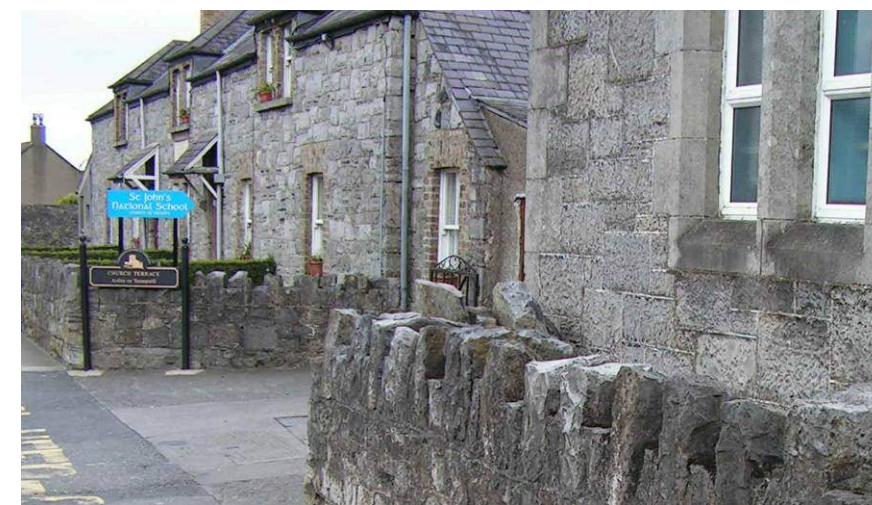
Fig. 3.6. A photograph of the almshouses with their brick lined openings on the left. A corner of the school building is shown on the right.
