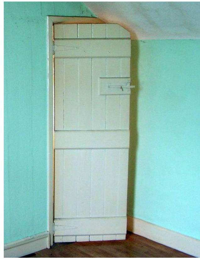
Fig. 7.13. A door at first floor level in number 3 Millview. (May 2011)
