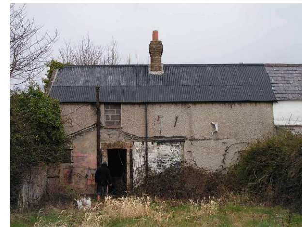
Fig. 6.7. The back of 1 Millview Terrace. The traces of the outline for the roof of the former extension can be seen on the rere façade. (June 2013)
