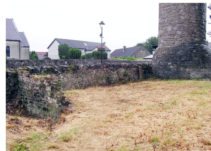
Fig. 4.69. A photograph of the boundary wall to the north of the round tower. Note the two stubs of wall immediately to the north of the tower and the remains of a boundary wall in the left foreground (June 2013)
