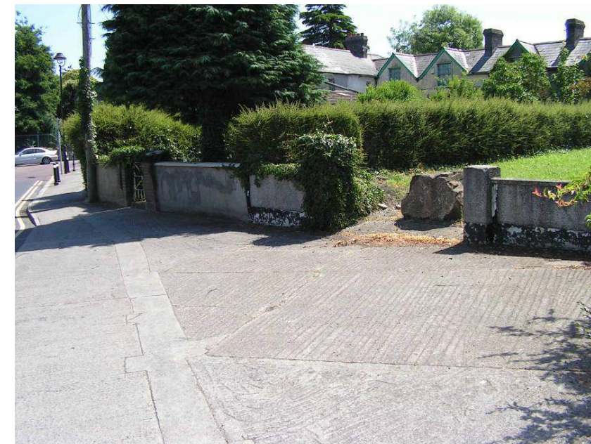
Fig. 15.1. The existing rendered brick boundary wall at the front or northern boundary of number 1 Millview Terrace. (July 2013)
