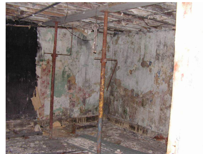
Fig. 8.6. Temporary propping of the floor in 1 Millview Terrace. (March 2013)
