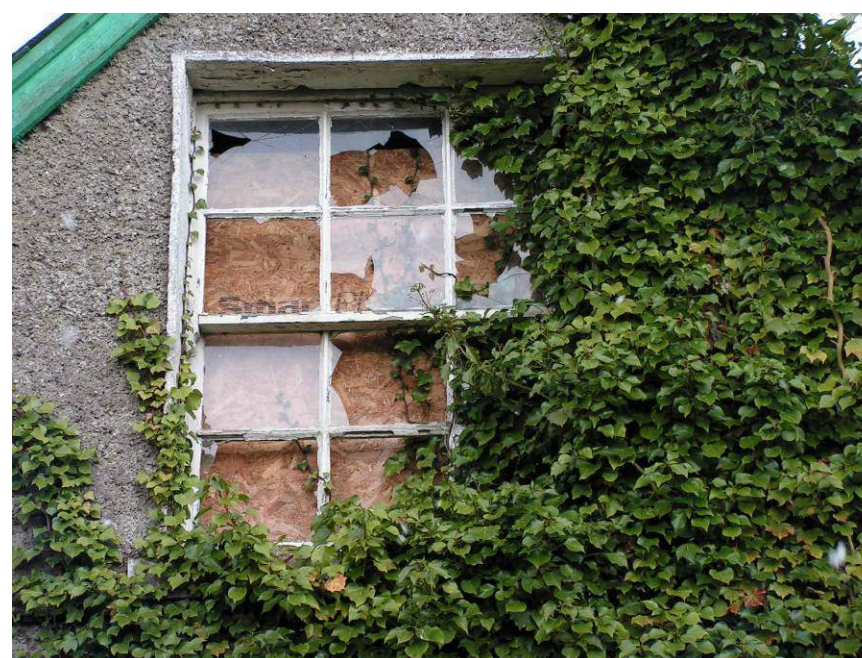
Fig. 7.6. 2 Millview Terrace. A closer view of one of the windows (March 2013)
