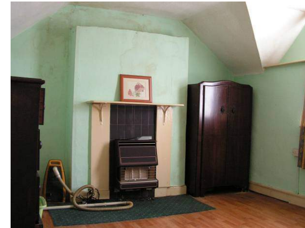
Fig. 6.22. The westernmost bedroom of 3 Millview Terrace (May 2011)
