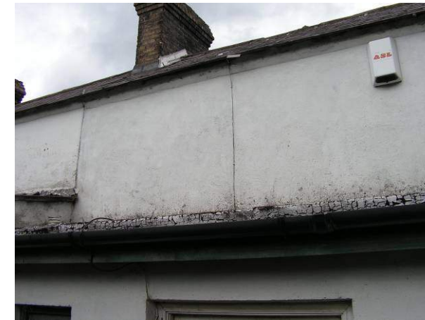
Fig. 6.21. The rear extension to 3 Millview Terrace (January 2013)
