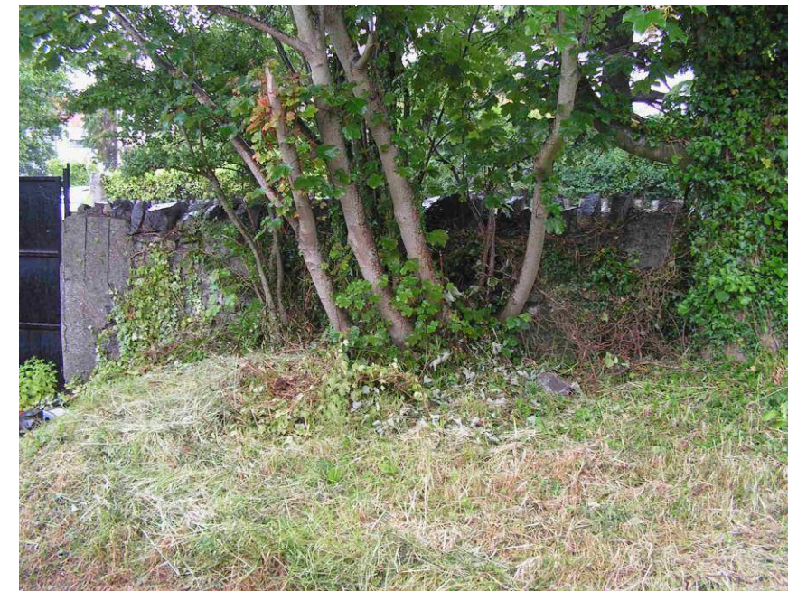
Fig. 7.2. The northern end of the same stone boundary wall along Tower Road, just to the south of the gate beside 15 Tower Road. (June 2013)
