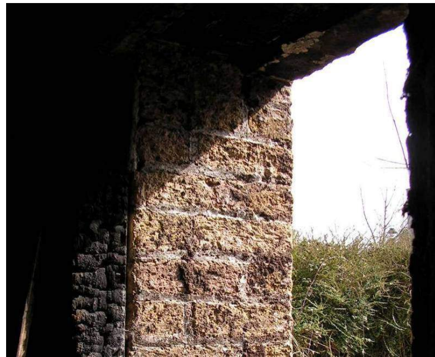
Fig. 3.1. The brick reveals at the back door of the house of 1 Millview Terrace. These were exposed after the building was damaged by fire; a charred door frame is visible on the left side of the photograph
