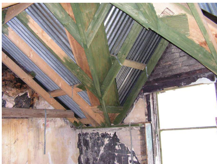
Fig. 8.4. The new roof of 1 Millview Terrace, installed after the houses was severely fire-damaged. (March 2013)
