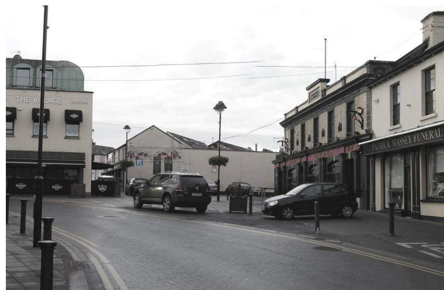
Fig. 4.66. The same view as Fig. 4.64, January 2013. The long blank wall was once behind a row of small houses which were laid along the long vacant site beyond "Quinlan's public house, a.k.a. The Black Lion".
