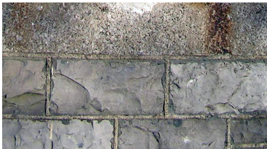
Fig. 3.7 A close up view of the front façade of Clondalkin library (1911). The rock-faced calp limestone contrasts well with the granite cill above.
