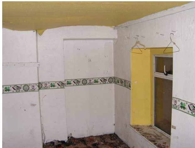
Fig. 6.17. First floor room with blocked up fireplace in the party wall of 16 Tower Road. (January 2013)
