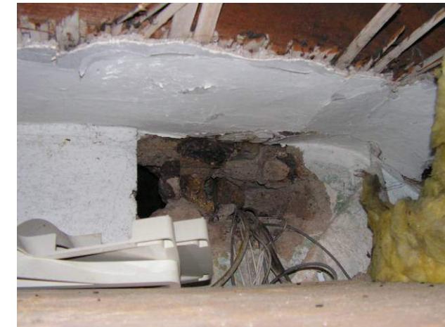
Fig. 6.30. The attic above 15 Tower Road. A fragment of the older plaster and lathe ceiling remains above the modern plasterboard ceiling on the bottom of the photo. The artificial roof slate above has been laid on a bituminous felt.
