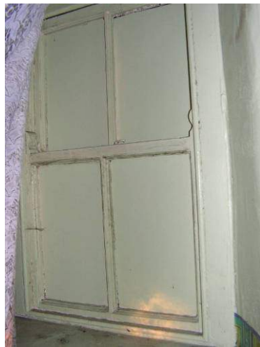
Fig. 6.18. 16 Tower Road: blocked up sash window in the rear facade
