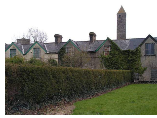
Fig. 6.8. The fronts of 3 and 2 Millview Terrace (left to right) (June 2013)
