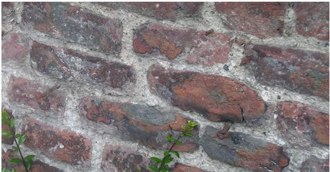
Figure 3.9. A close up view of the former kitchen garden wall: a wrought iron pin in the mortar joint of part of the wall which would have once secured old rags to retain a soft fruit tree espaliered to the wall.
