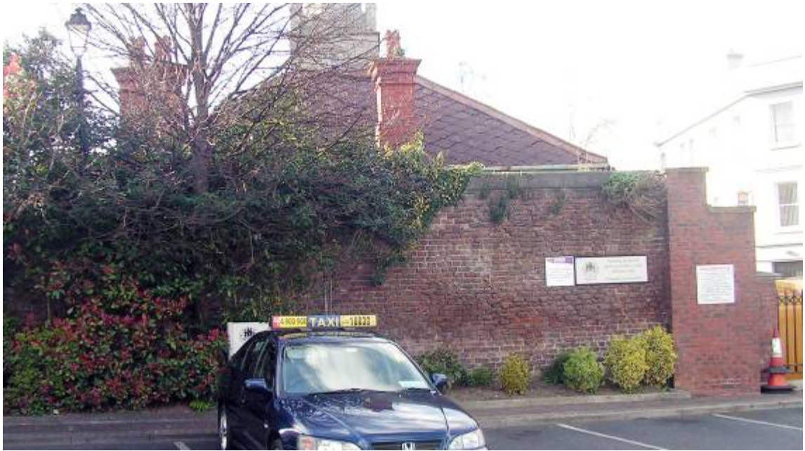
Figure 3.8. The brick-facing (probably late seventeenth or early eighteenth century) to an older calp limestone demesne wall of the former kitchen garden behind the former Court of Petty Session (1914). The high brick wall retained solar heat and provided a sheltered environment for growing soft fruit.
